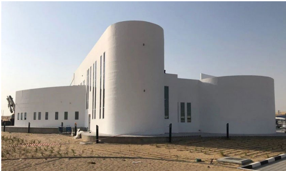
Figure 11: Apis Cor's finished structure, the largest 3D-printed building in the world 3
