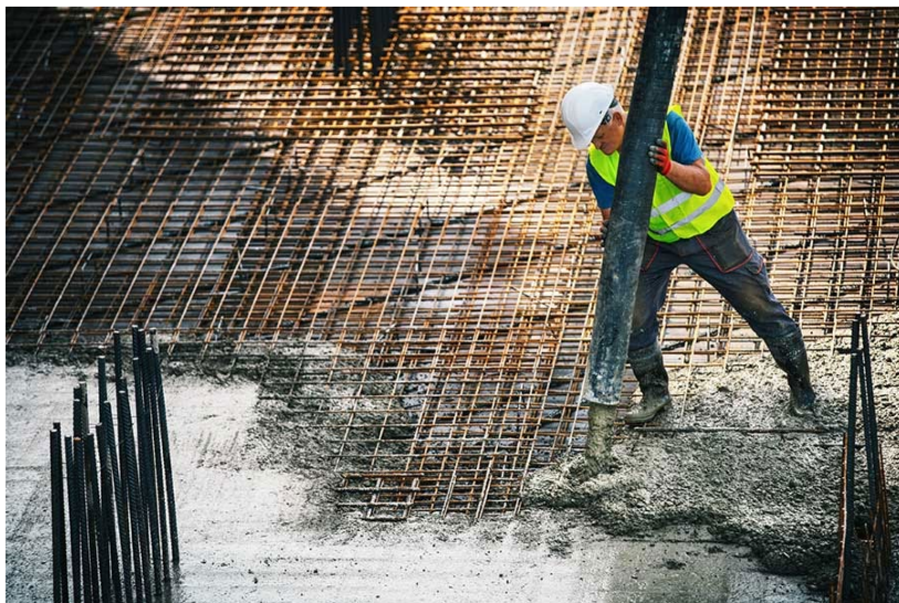
Figure 1: Concrete being poured by a worker 3
