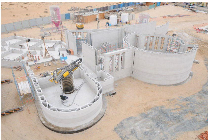
Figure 10: Apis Cor's building site, Dubai, with 3D printer mid construction 4
