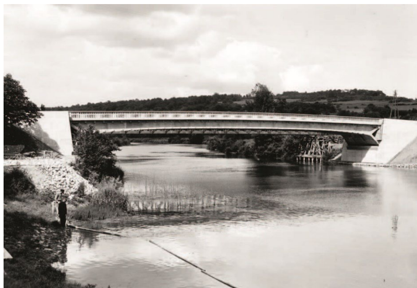
Figure 5: One of the earliest prestressed concrete bridges, designed by Eugène Freyssinet, completed in 1946, spanning 55 metres 1
